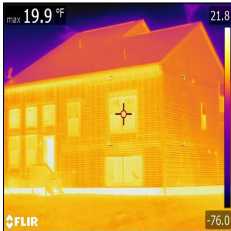
No Exterior Continuous Insulation
